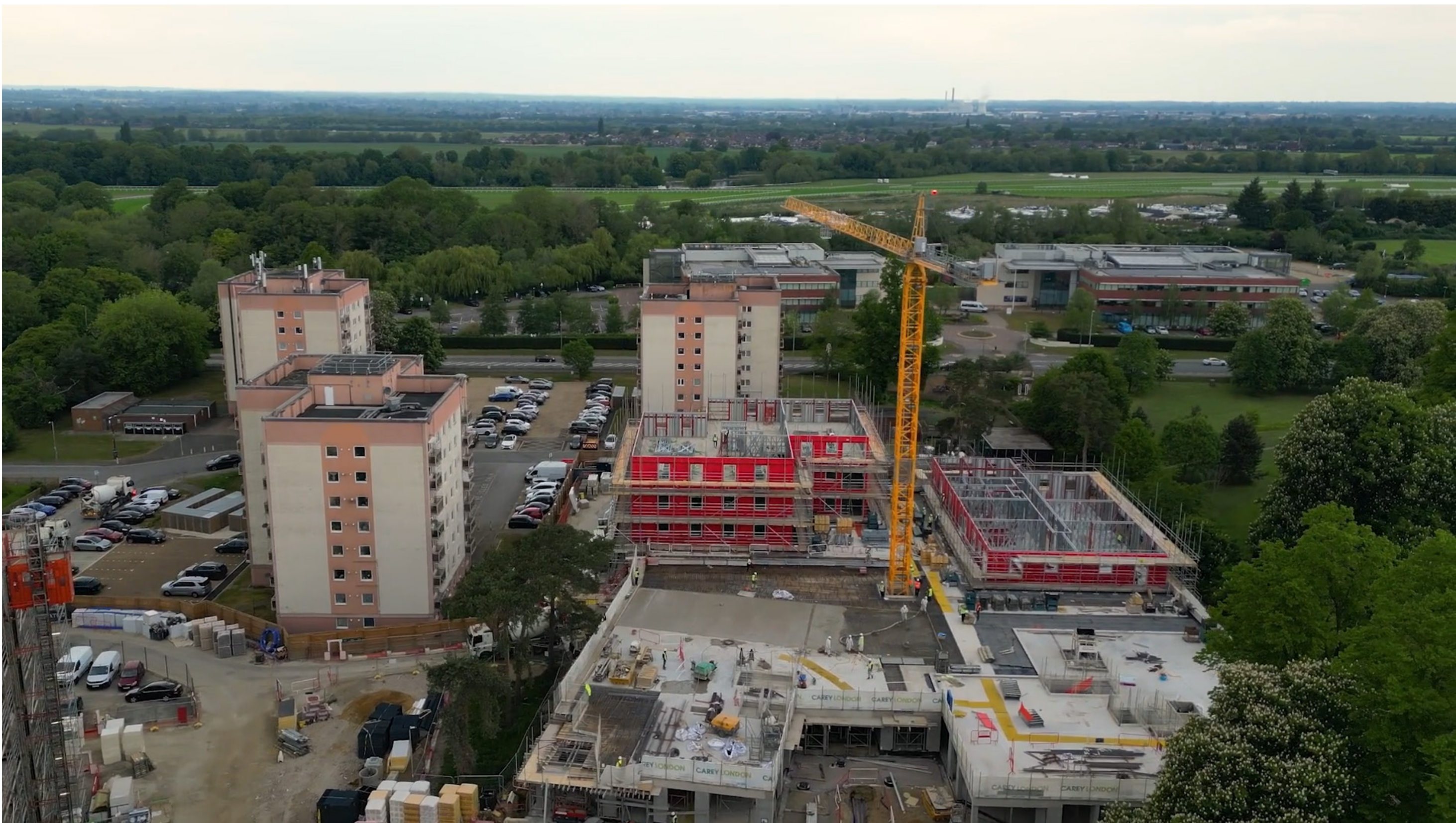
Drone aerial photo of Plot C under construction
