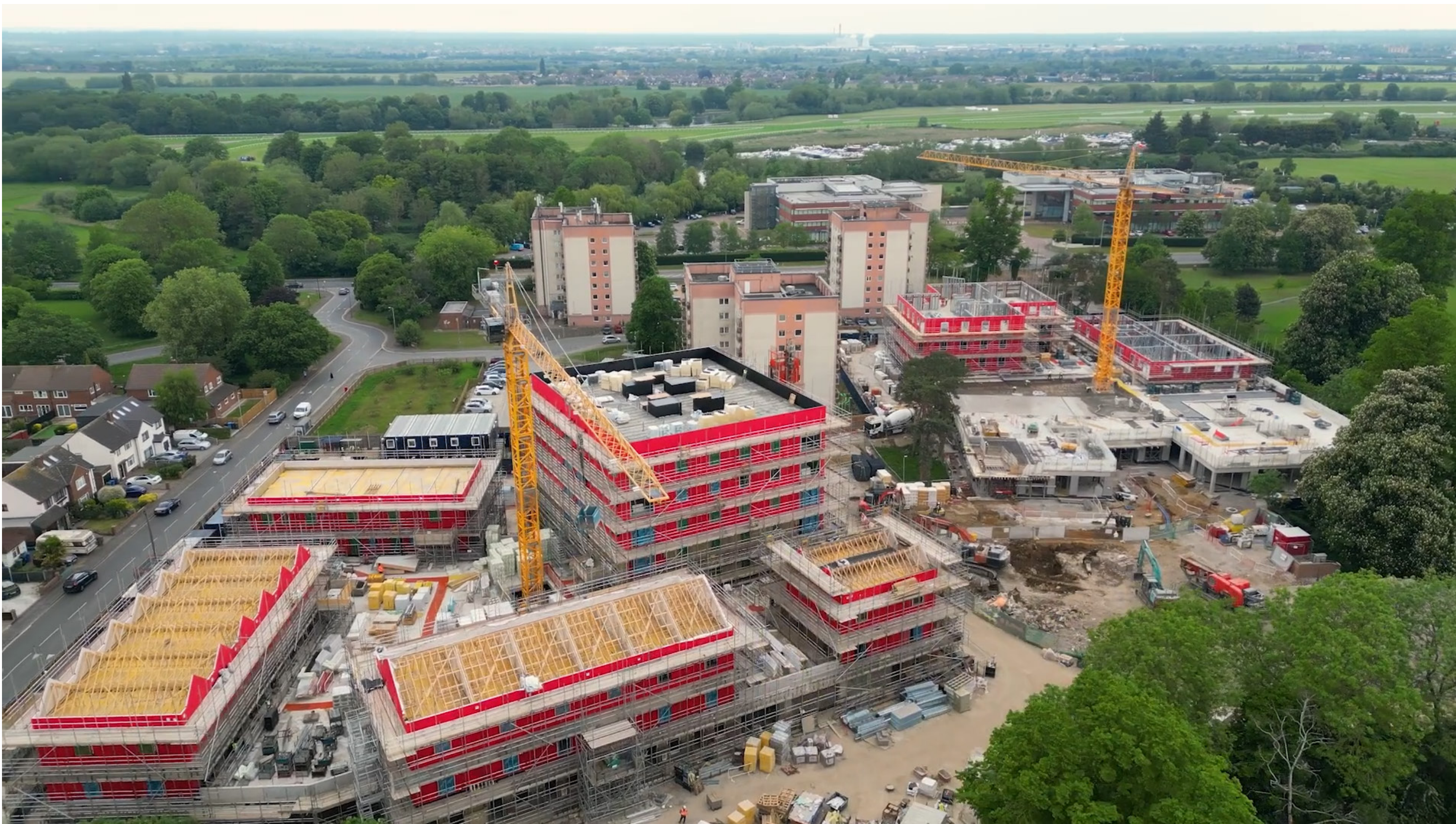
Drone aerial photo of Plot D under construction
